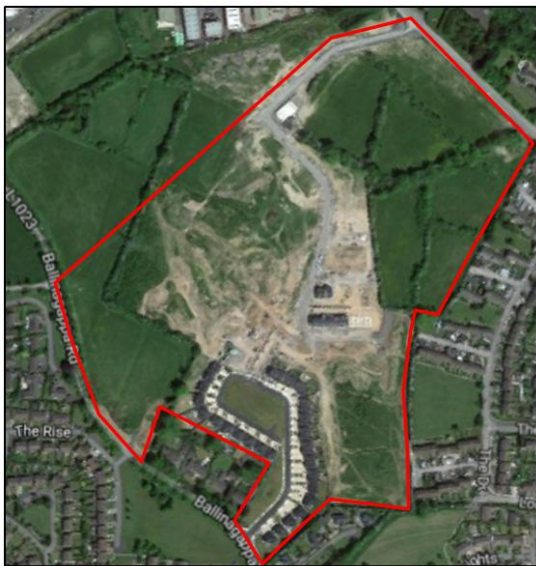
Figure 12.4(a): KDA 3 Aerial View
